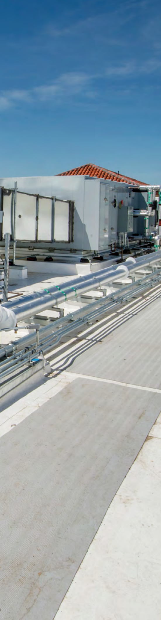
Rooftop HVAC Installation
